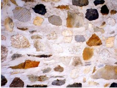
Rather than doing freehand stonework with a trowel and level, stones were placed with a good face against boxed formwork, and the space behind them was filled with concrete, making a beautiful hybrid wall of stone and concrete. Buildings constructed with this method are structurally sound and long-lasting, while requiring little maintenance.
